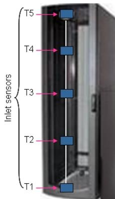
**Figure 2. Rack Inlet Temperature Sensors**
