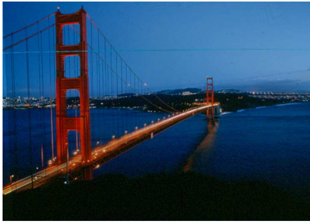
(a) Image with defects
